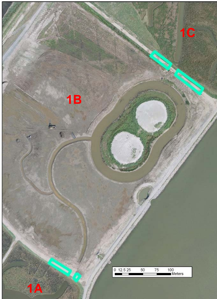
Figure 5. Aerial photo of the cross dikes between Cells 1A/B and 1B/C (before cross dike breach) highlighting potential nesting areas that could be expanded and maintained vegetation free with minimal danger of erosion.
